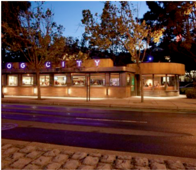
The new façade.
